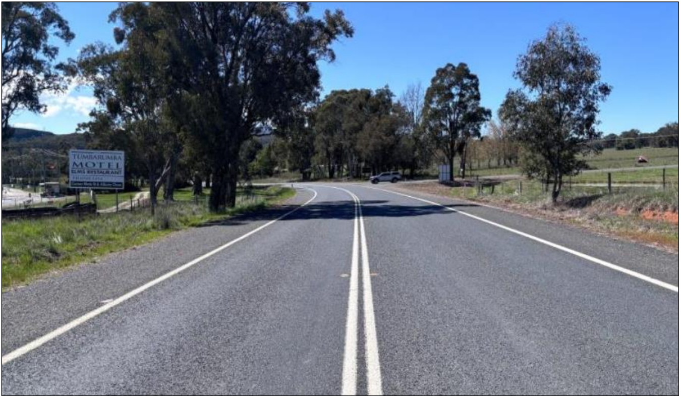
Figure 5: Jingellic Road facing east on approach to Corundum Road
