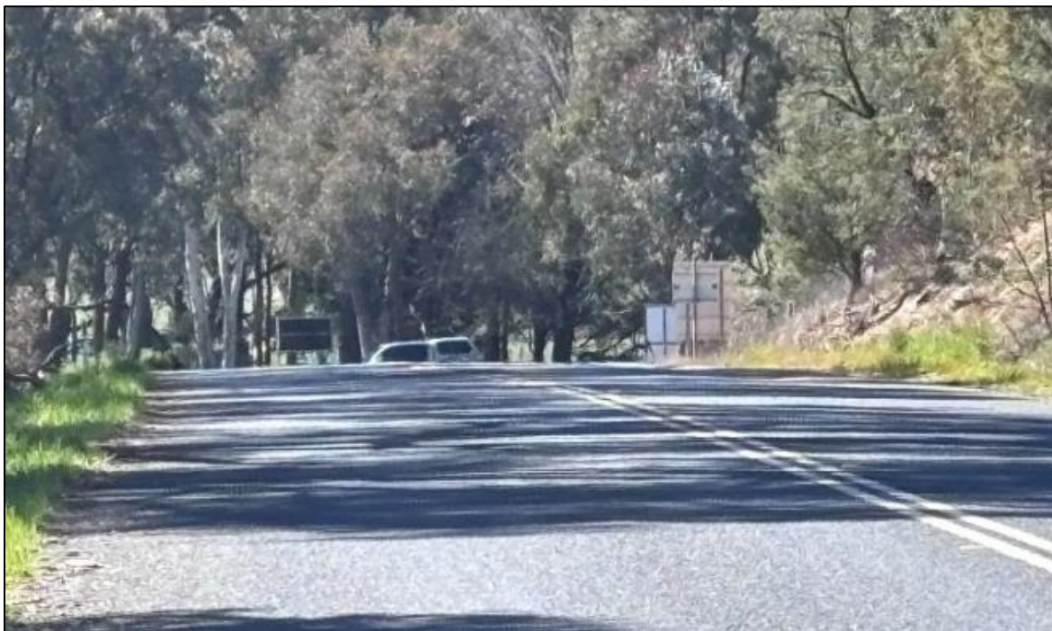
Figure 14: Crest (1.5% downgrade) restricting available sight distance of 290 m on approach to Corundum Road from the south
